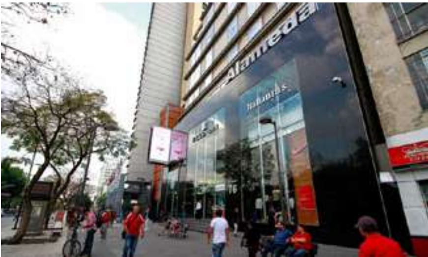
Parque Alameda In the heart of historic downtown Mexico City facing the majestic Palacio de Bellas Artes. 15,825 m² of leasable area 302 parking spaces
