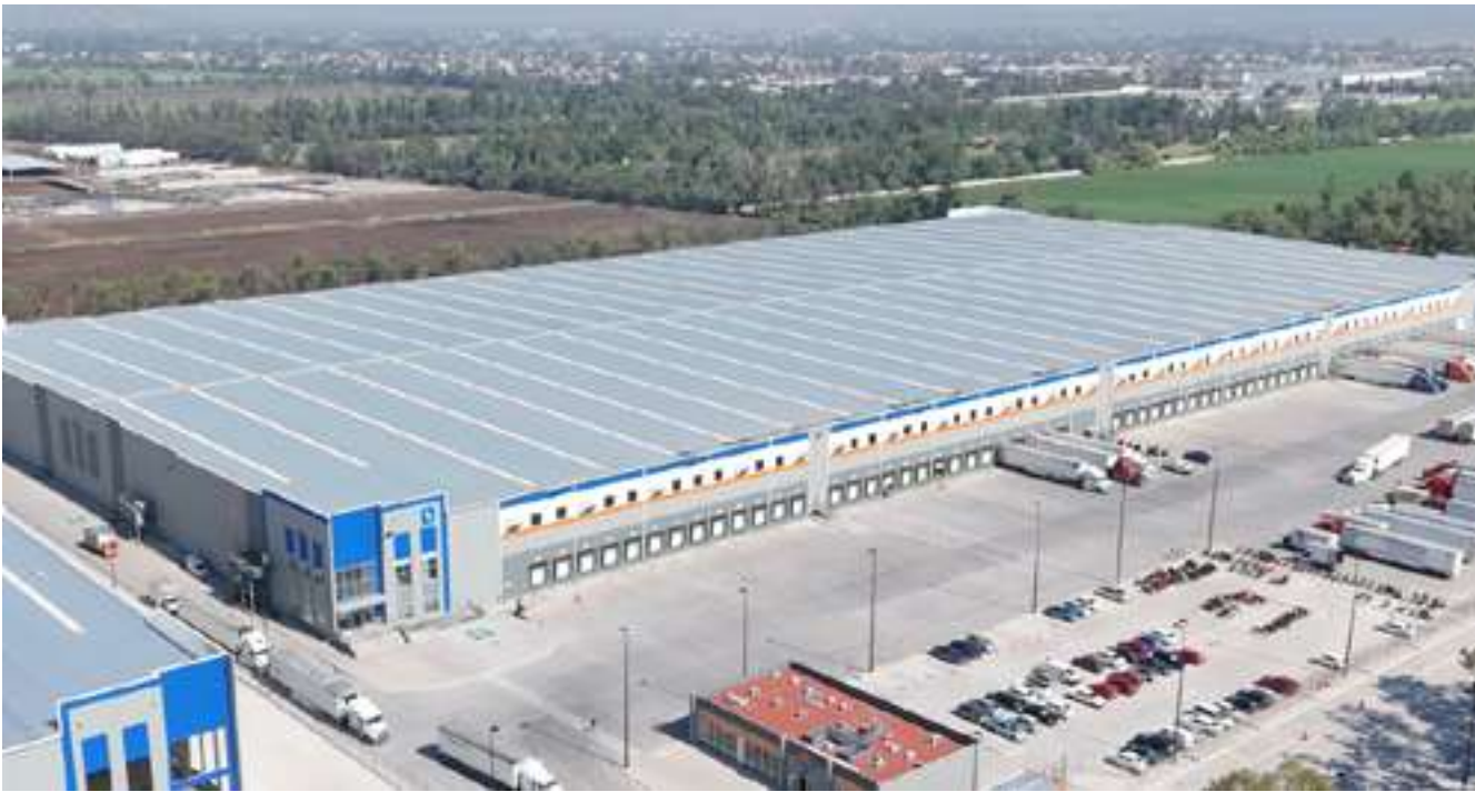
Parque Industrial Danhos Palomas, Phase I A build-to-suit development with triple-A specifications, designed to hold the distribution center for a leading supermarket chain. The project is located in Cuautitlán, Mexico State, and was completed and delivered in 2025. 52,182 m² of leasable area
